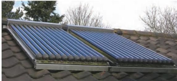
**ON SUNNY DAYS**, the solar tank provides hot water for the whole house with temperatures reaching 70°C or higher from around mid morning until the end of the day. During the night, the water remains warm enough to be used for the washing machine. On very cloudy days, water from the solar tank may only reach 25°C and so will be fed into the main boiler tank. Even in this east-facing property, where hot water from the solar system cannot be stored, the benefits have been noticeable.
