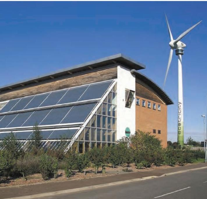
**THE MOST IMPRESSIVE** visitor attraction is the Enercon E-66 wind turbine with a unique viewing platform located just under the hub. In 1999 it was the UK's first multi-megawatt wind turbine and one of a new generation of direct drive, variable speed wind turbines brought to the UK by Ecotricity. A second turbine was opened in July 2003.
